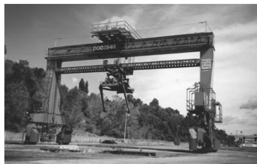
Fig. 40 t gantry crane
